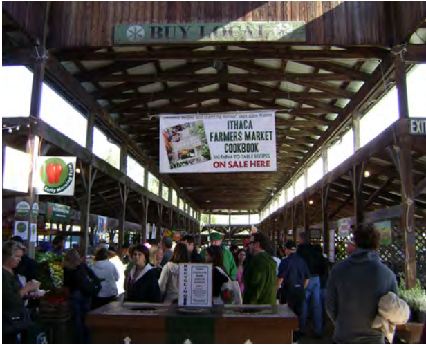
Stepped roof heights at Ithaca Farmers Market, Ithaca, NY. Photo courtesy Alana Mautone ( http://ramblinwitham.blogspot.com/2011/10/ithaca-ny-farmers-market-buying-local.html ).
