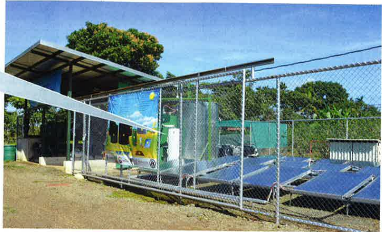
The solar-biopower unit includes a 32 m 2 solar thermal panel (above), a 20 m 3 digester and a 50 m 3 biogas storage bag (close up of digester and storage bag on left). One metric ton/day of poultry and cattle manure and food waste is processed.
