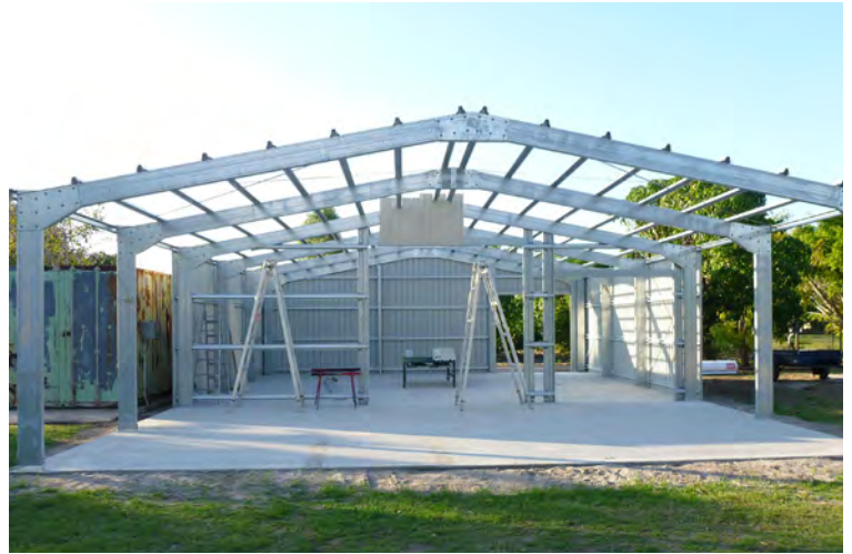
Prefabricated steel structure. Jensen Shed by WAZ Steel and Sheds, Queensland. Photo courtesy of WAZ Steel and Sheds ( http://steelandsheds.com.au/jensen-shed-photos/4576223477 ).
