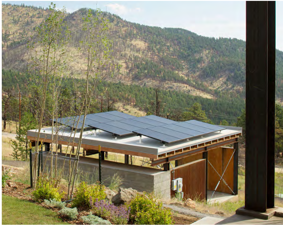
Carport with solar panels, Sunshine Canyon House, Boulder, Colorado, designed by Renée del Gaudio Architecture. Photo courtesy David Lauer, ©2013 David Lauer Photography.
