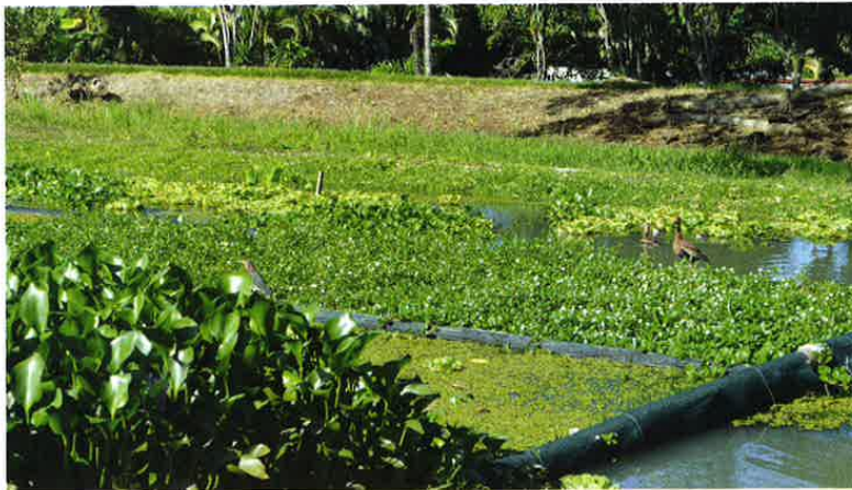
Effluent (filtrate) from the digester is treated in a wetland with some vegetation and two open surface filters with floating plants and vegetative mats.
