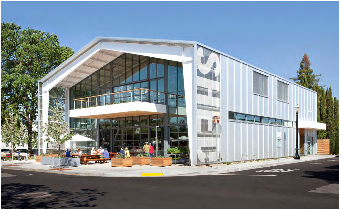
Prefabricated metal structure and modern interpretation of barn typology. Shed Store and Cafe, Healdsburg, by Jensen Architects. Photo by Mariko Reed, courtesy Jensen Architects ( http://jensen-architects.com/our_work/featured_projects ).
